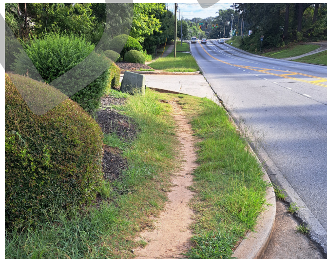
MISSING SIDEWALK ON WEST SIDE OF ROAD BETWEEN DRIVEWAYS
