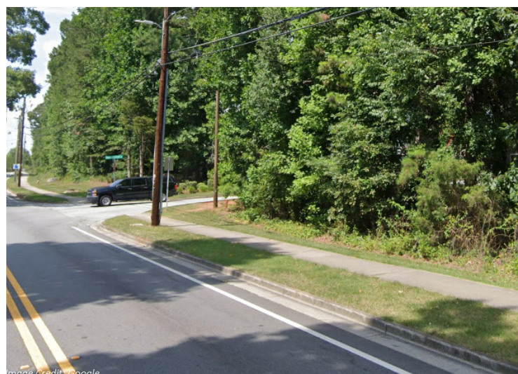
UTILITY POLES CLOSE TO CURB NEAR STONEBRIDGE CREEK LANE MAY NEED TO BE RELOCATED
