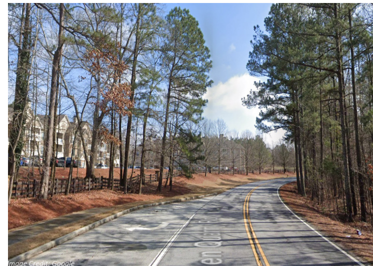
SIDEWALK ENDS EAST OF WESLEY PROVIDENCE APARTMENTS
