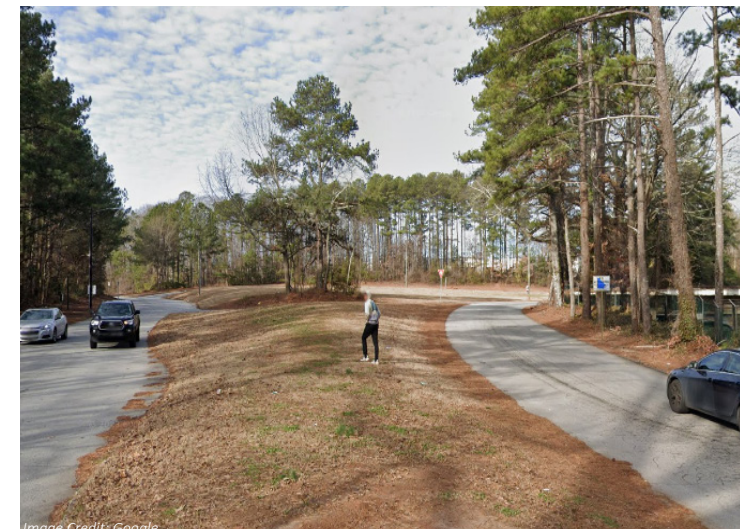
GAP IN SIDEWALK ACROSS INTERSECTION AT FAIRINGTON PARKWAY AND RUE FONTAINE
