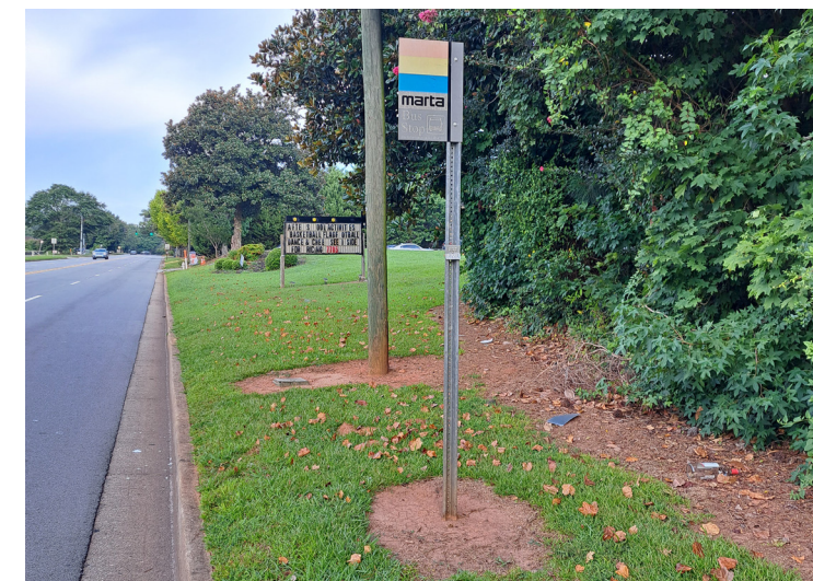
BUS STOP WITH NO CONNECTING SIDEWALK OR WAITING AREA
