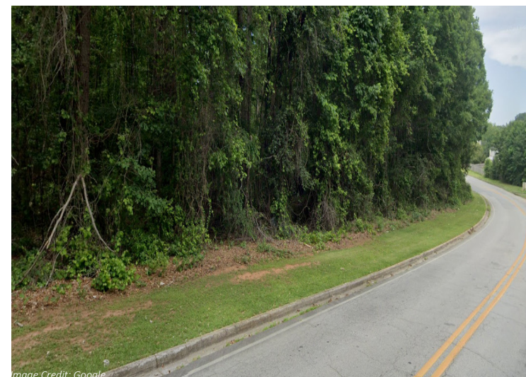
DESIRE PATHS AND OVERGROWN VEGETATION ALONG NORTH SIDE OF ROAD
