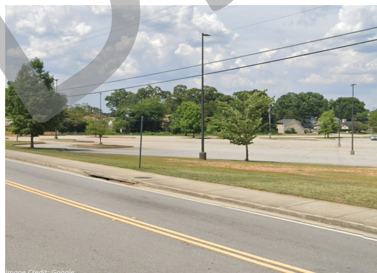
OPPORTUNITY TO EXPAND SIDEWALK TO SHARED-USE PATH IN FRONT OF HIGH SCHOOL
