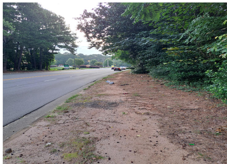
MISSING SIDEWALK AND DESIRE PATHS, WEST OF PANOLA ROAD ON SOUTH SIDE
