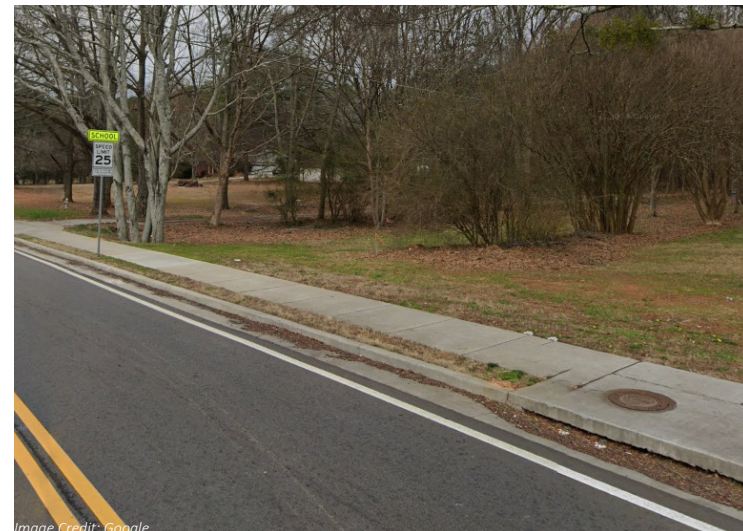
THERE IS GENERALLY SUFFICIENT ROOM TO UPGRADE SIDEWALK TO SHARED-USE PATH
