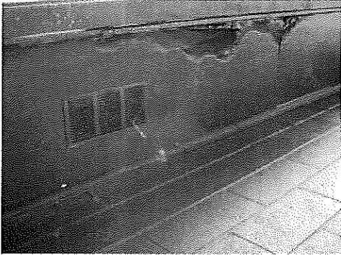
Soffit at Rear of Building
