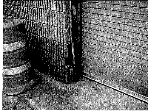
Repair CMU Wall
