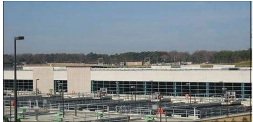
DeKalb County Water Treatment Plant
