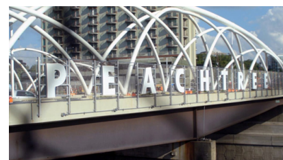
Figure 5-5: Peachtree Street Gateway Bridge over I-85
