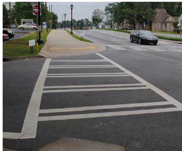
High-Visibility Crosswalk with Pedestrian Countdown Signal, Cobb County, GA
