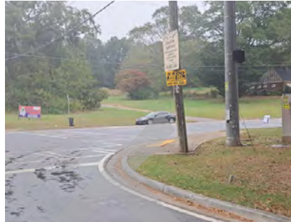
ADA Compliant Gaps Present on Southeast Corner of Intersection with Covington Hwy but No Sidewalks
