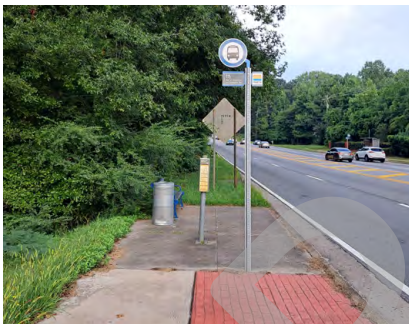
Dead-End Sidewalks Are Common Along Covington Hwy, Including West of a Bus Stop Across from Strathmoor Manor Dr
