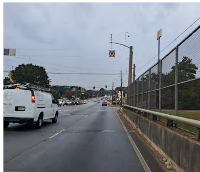
View North from Bridge over I-20; Sidewalk Only Present on West Side of Bridge and not East Side
