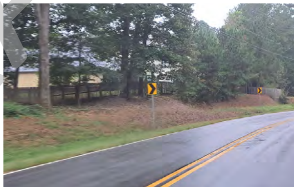
Tight Roadway Curvature and Necessary Drainage Improvements Make Adding Sidewalk Along Turner Hill Road Among the Most Complex Sidewalk Recommendations (SW-76)
