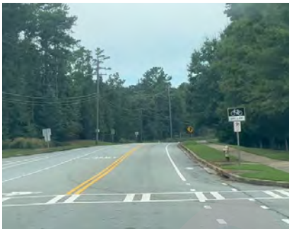
Existing Crosswalk and On-Street Bicycle Lane at Flat Rock Elementary School
