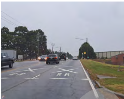
Four Travel Lanes between Covington Hwy and S Stone Mountain Lithonia Rd with Minimal Sidewalks and Railroad Crossing Between Tribble St and Marbut Rd
