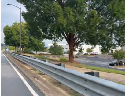
Guardrail Separates Sidewalk from Travel Lanes on north side of Mall Pkwy from Stonecrest Trce to Wesley Stonecrest Cir
