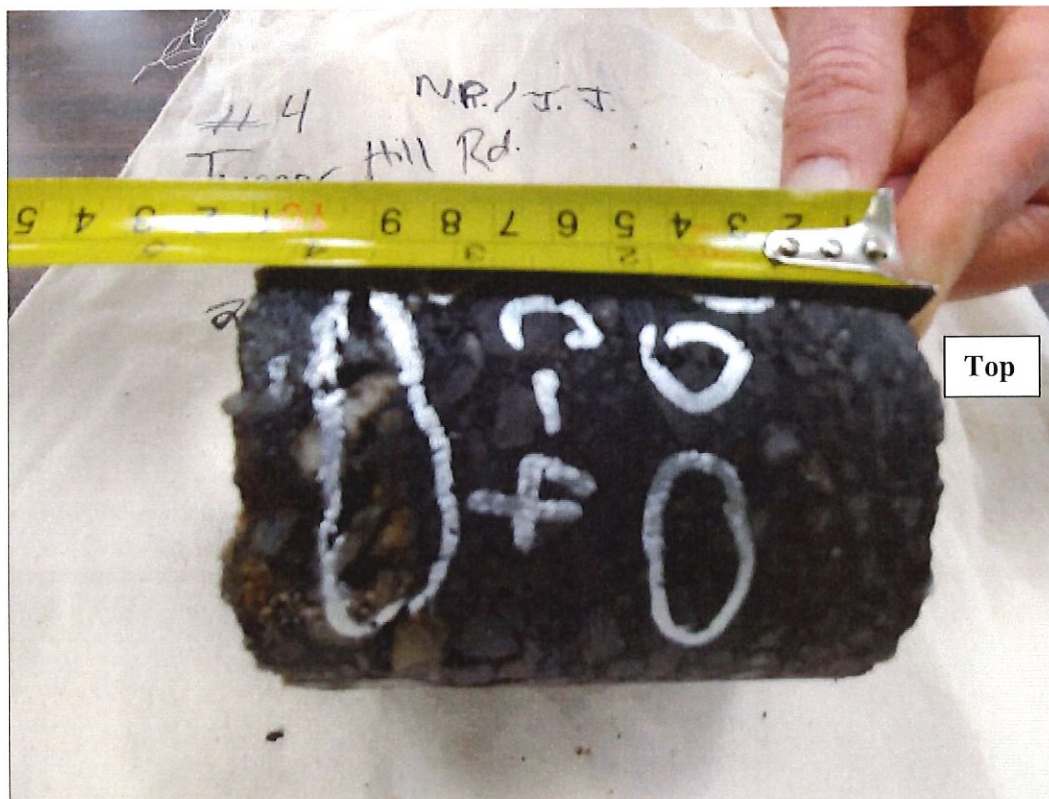
Core 4, Turner Hill Road, Station 45+80±, Northbound, Lane 1, 8.0' Left
