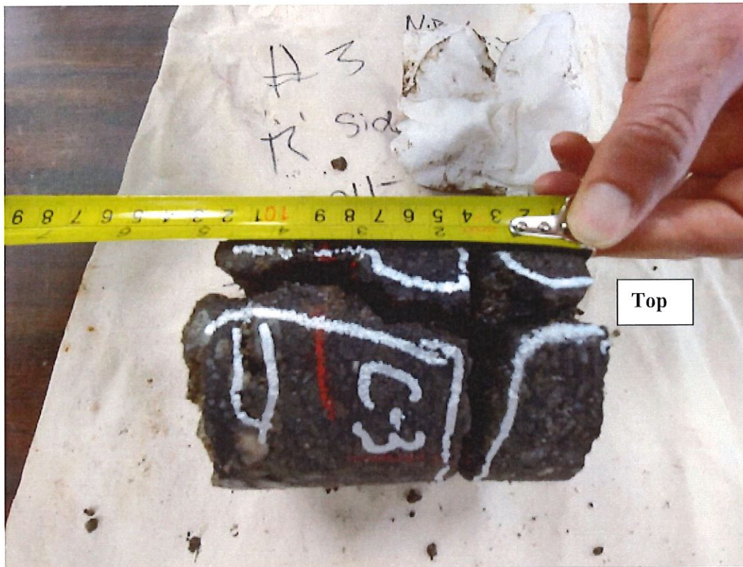
Core 3, Turner Hill Road, Station 40+40±, Southbound, Lane 1, 8.5' Right
